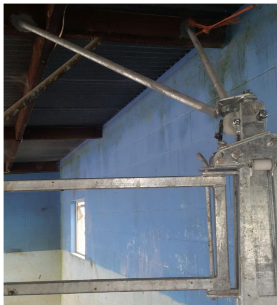
Figs 10 & 11. Post Diagonal supports
