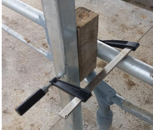
Fig 9. Post clamped in position
