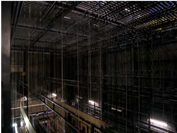
A typical counterweight flying system
