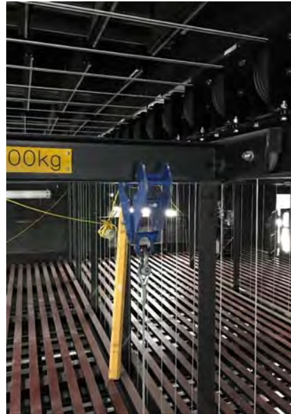
Example of a travelling beam with accessories
