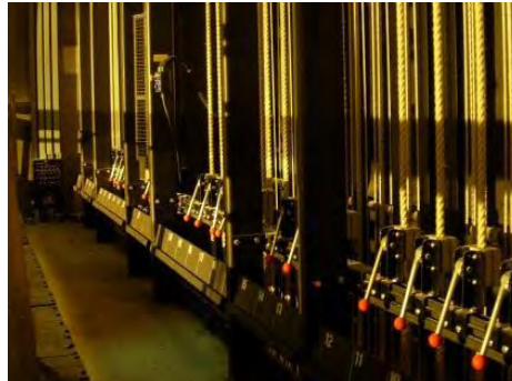
A typical counterweight flying system
