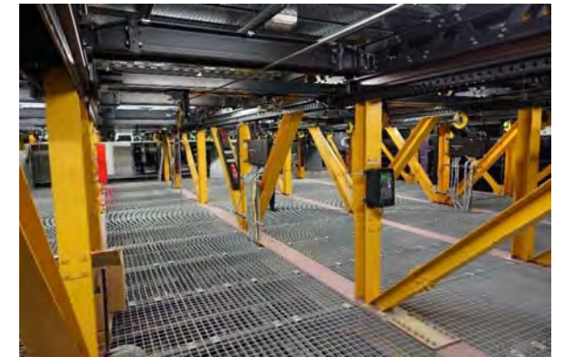
Example of steel mesh grating installed in a venue with flying lines below the grid
