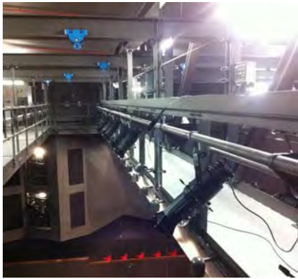
Example catwalks with outriggered equipment bar
