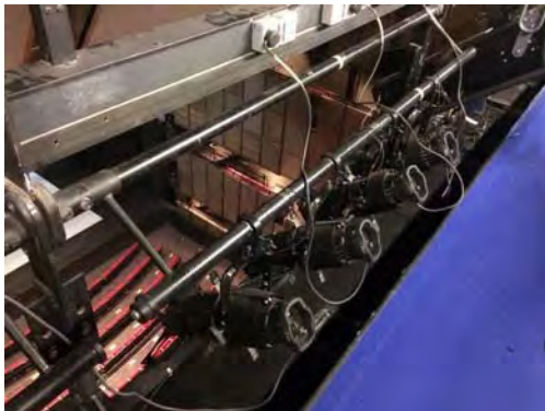
Example lighting bar fixed back from catwalk edge
