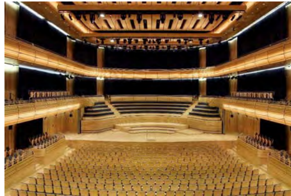
Variable acoustics curtains deployed on the walls, Sage Gateshead, UK
