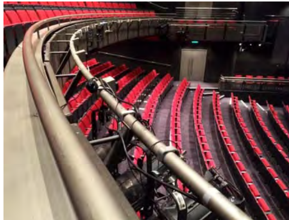
Example of a balcony front fixed equipment rail
